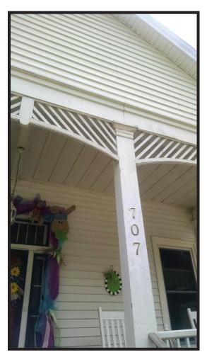
Figure 14. Porch Detail Showing Square Post and Matchstick Frieze
